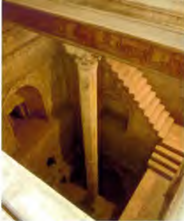
The nilometer in Rawada Island at Fustat, near Cairo, completed in 801-802 CE. The octagonal column in the centre is used to measure the height of the water in the Nile in cubits.
